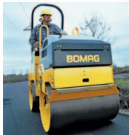
BW90AD-2 in action on an asphalt repair
