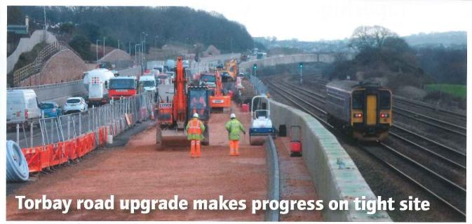
With a busy highway to one side and a railway on the other contractors building the South Devon Link Road make good progress widening part of the A380 between Newton Abbot and Torquay. The 1km on line improvement will then join up with a new 5km bypass of the village of Kingskerswell.
