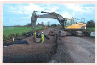
**LIFELINE FOR FLOOD PRONE VILLAGE:** Raising of a 500m stretch of road near the Somerset village of Muchelney to help keep the highway open during major floods has almost completed. The project is designed to allow continued access to and from Muchelney, which was cut off last winter.
