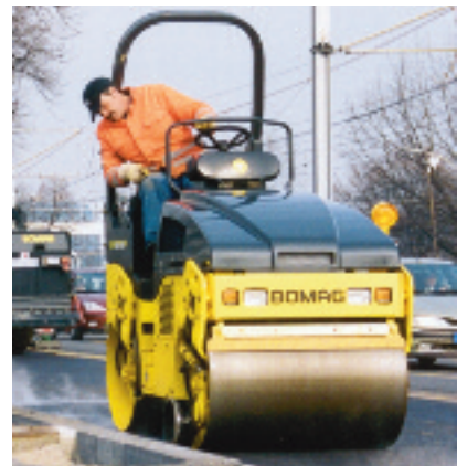
BW100AD-4 rolling a curbline.
