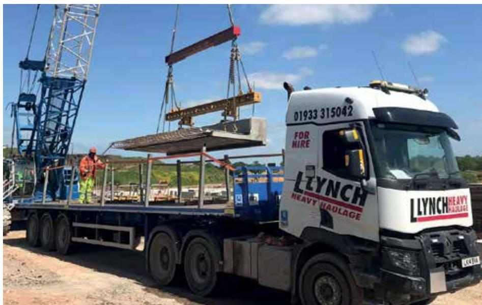
The precast slabs are being used instead of an in-situ build to ensure a much higher quality finish, as well as providing a safer working process.
